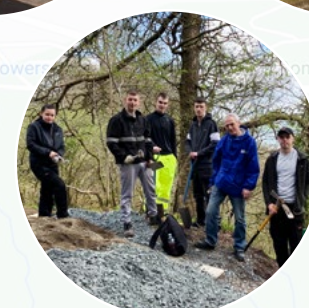
Trainees, employed by Inverclyde Trust, continue restoration work on The Glen
